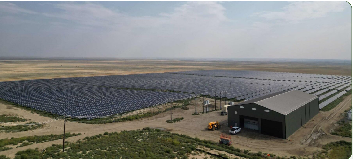
SOURCE: Elemental Energy ( https://elementalenergy.ca/project/chappice-lake-solar-storage/ )
